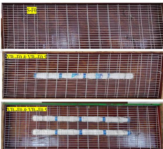
Fig. 2. Fabrication of ferrocement slabs.
