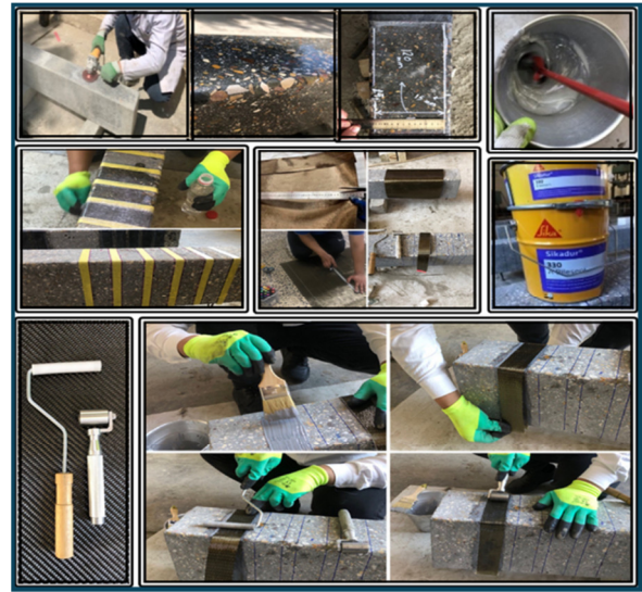
Fig. 2. Enhancing concrete: bonding BFRP sheets for strengthening.
