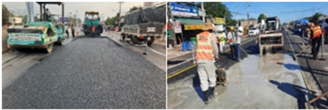
Fig. 2. The construction process of the SFC layer.
