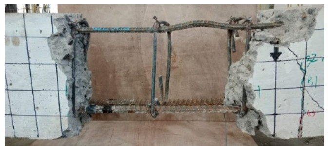
Fig. 12. Residual condition of beam specimen HCB-1.
