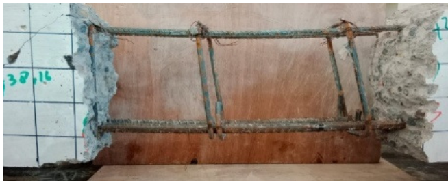
Fig. 14. Residual condition of beam specimen LCB-1.
