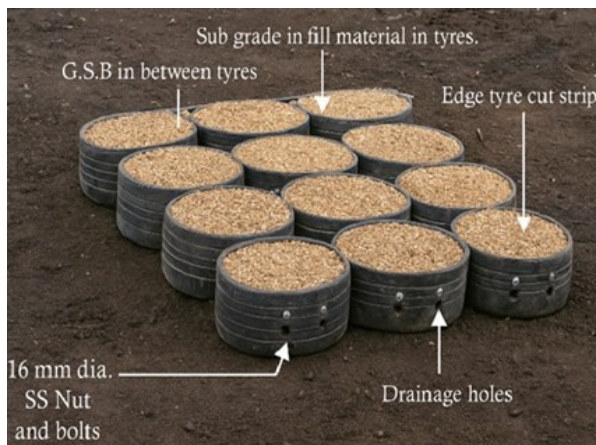
Fig. 1. Honeycomb grid structures of geo-tires.
