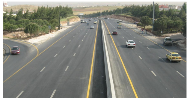
Fig. 1. Test section on Queen Alia international airport highway
