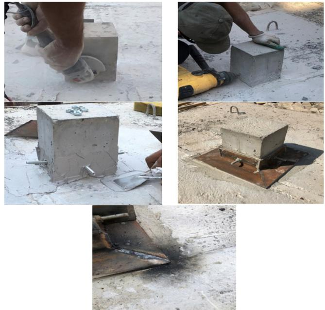
Fig. 6. The strengthening steps of column-slab connection.
