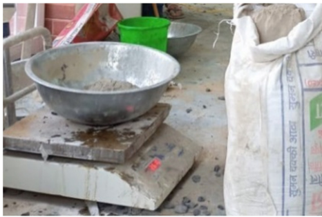
Fig. 2. Preparation of dry mix.
