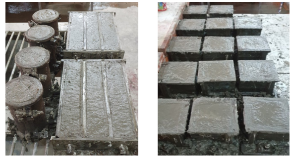
Fig. 2. Casting concrete molds.
