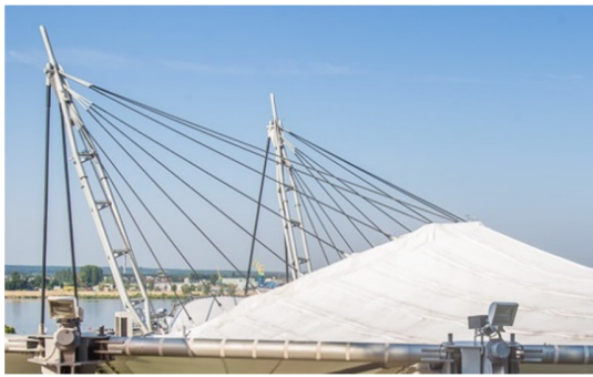
Fig. 1. The considered amphitheater's roof with pylons, Poland.
