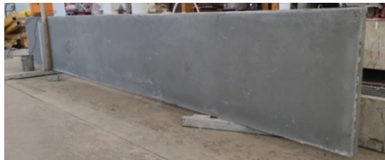
Fig. 3. UHPC plate after removing the formwork.
