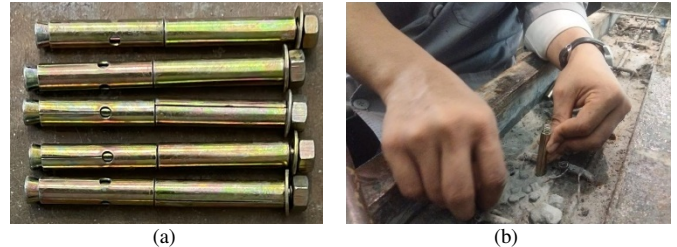
Fig. 2. (a) Dyna-bold anchors, (b) installation.
